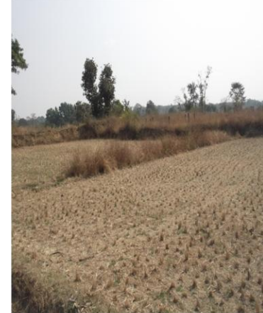
Land Leveling activity
