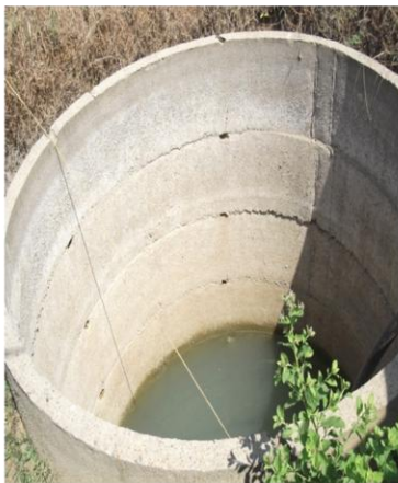
Dug well built
