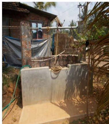
Dug well built
