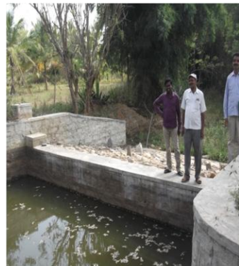
Check Dam built
