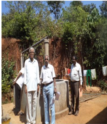
Dug well built
