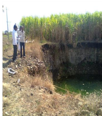
Dug well excavated
