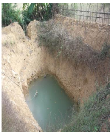
Dug well excavated
