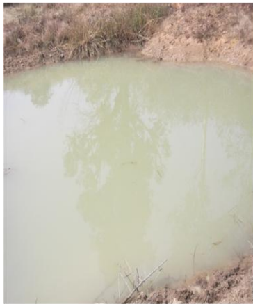
Dug well built
