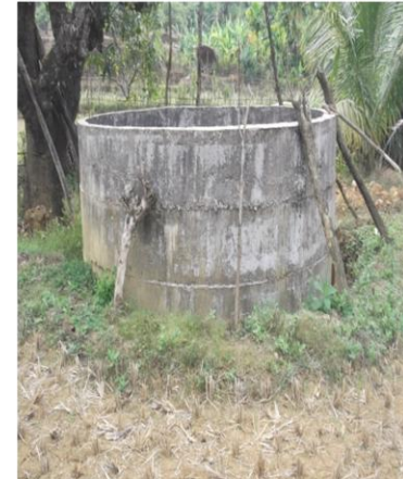
Dug well built
